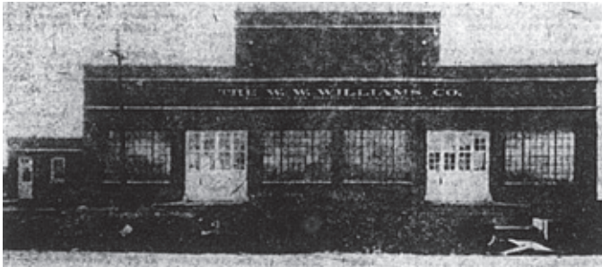
Original WWW building on Goodale in 1920.
