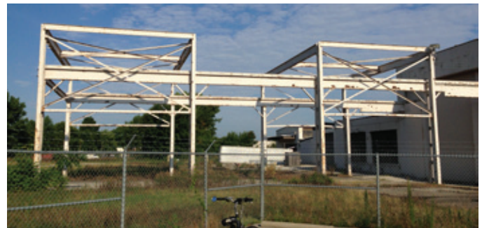
Crane support in back of WWW building; the crane extended to a private railroad spur.
