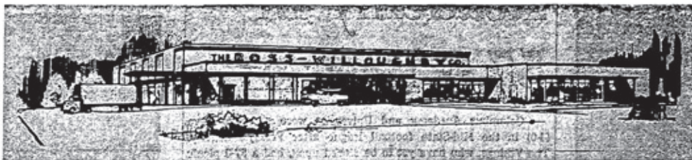
R-W Headquarters on Goodale Boulevard opened in 1955.
