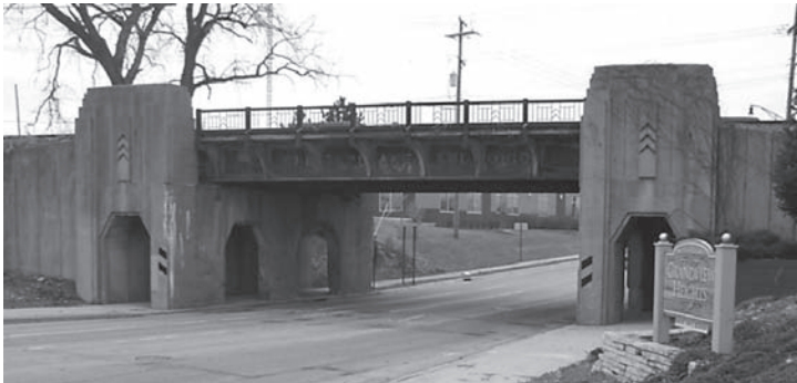
Goodale and 1938 Chesapeake and Ohio railroad bridge form southeast entrance to Grandview Heights.
