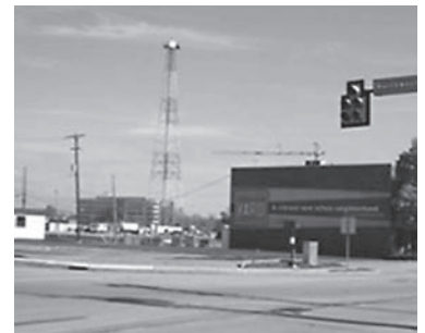
Grandview Yard construction in 2015 on site of former Big Bear warehouse on Goodale.
