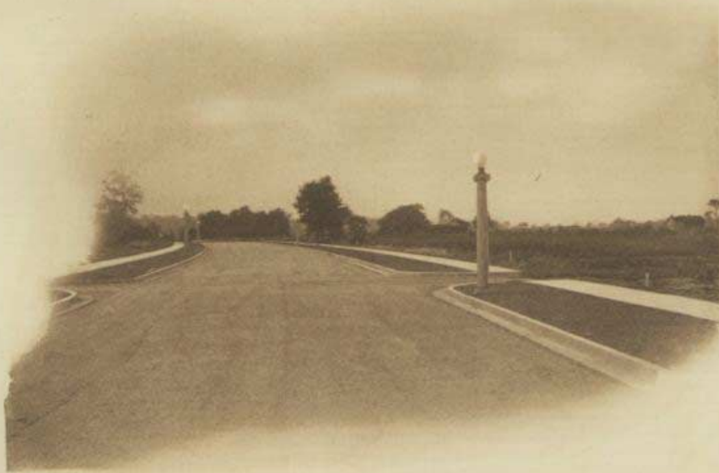
Typical Street in Upper Arlington nearing completion. Note symmetrical curve
