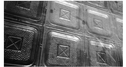
Tin ceiling tiles were retained by current Grandview Café owner.
