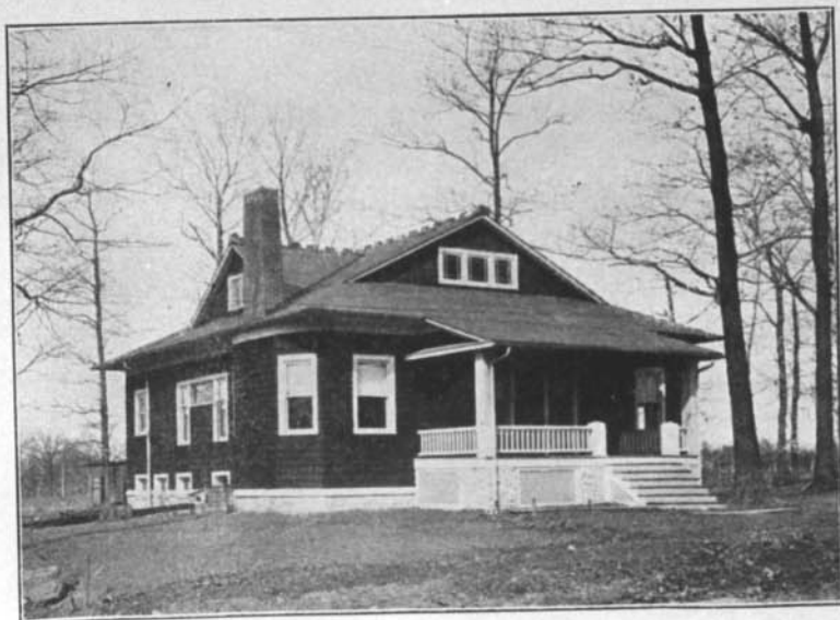
Residence of Mr. A. L. Frey, Paul Avenue
